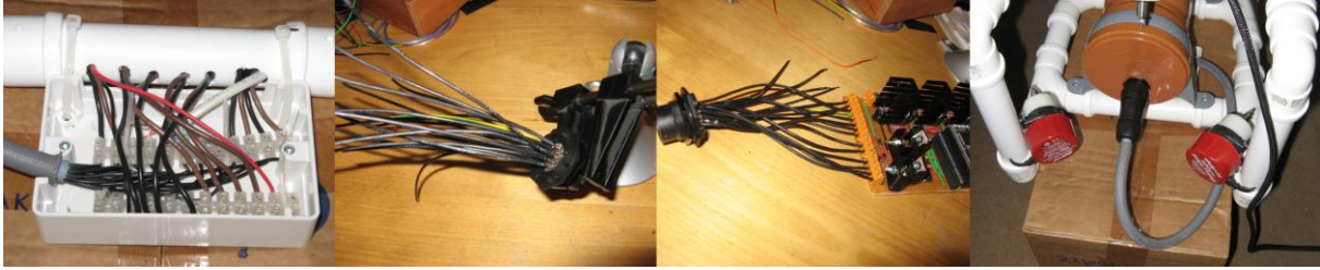
Figure 3.6. Construction of the 18-way cable and connectors.
